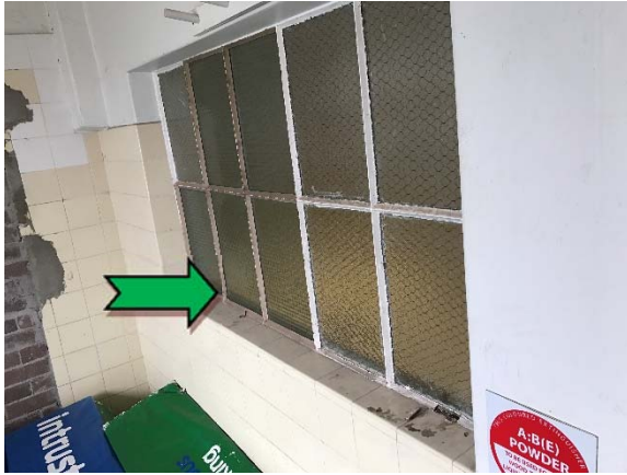
Photo 1. Exterior, ground level, throughout – non asbestos-containing window caulking.
